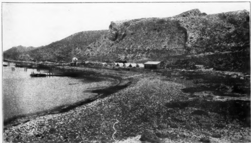
View Taken April 15, 1925, Before Any Work on Plant Had Started
